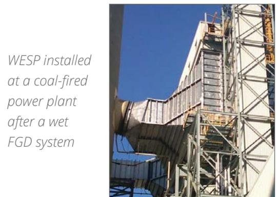
*WESP installed at a coal-fired power plant after a wet FGD system*
