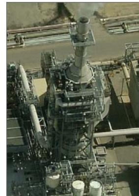
*WESP on top of wet scrubber on a refinery FCCU*
